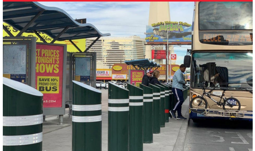
Bus Stop with Safety Bollards
